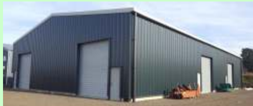
Newly Constructed 4,000 sq ft Workshop, Tysoe.
